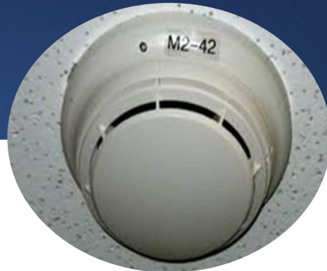
Typical Building Fire Alarm Smoke Detector
